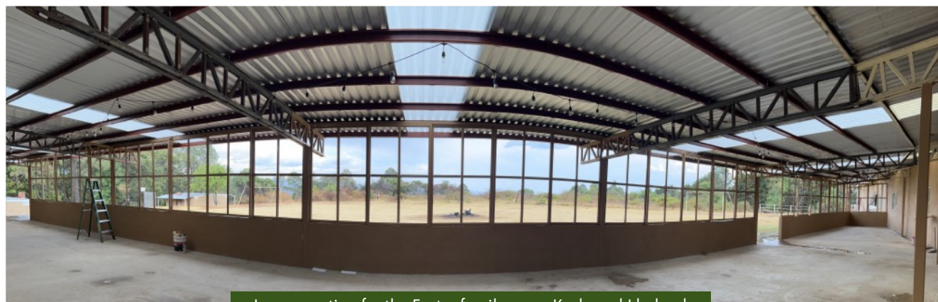
In preparation for the Easter family camp Keyla and I helped make these window frames for the new dining room extension.
