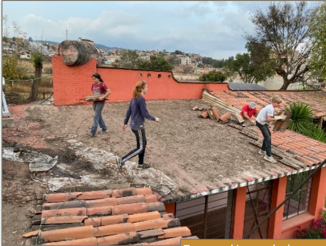
Team working on the huge project of re-sealing the leaky roof
