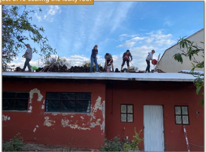
Team working on the huge project of re-sealing the leaky roof
